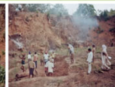
Villagers engaged for excavation of Raidiha Tank
