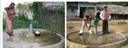
Tube-wells constructed under project in Burudanga and Siripur villages of Berhampur forest division
