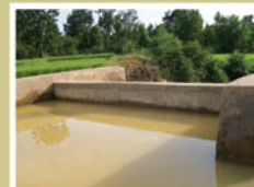
Check-dam in Beheramal village of Sambalpur (S) forest division
