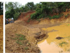
Renovated & partially filled tank
