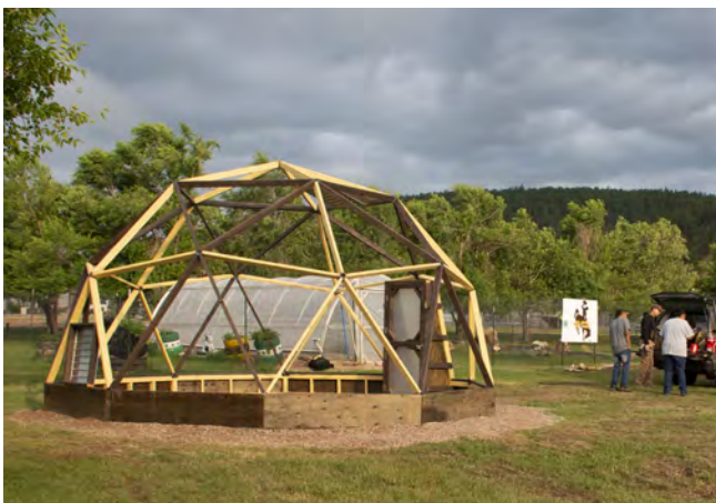
Building a geodesic dome, Sundance, Wyoming
