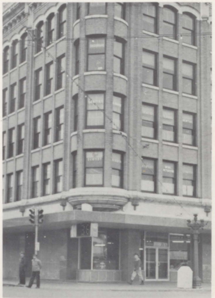
The newly remodeled FIRST NATIONAL BANK of Virginia is always ready to give you the finest in banking service.
