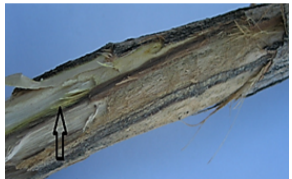
Figure 3: Yellowish discoloration of the wood surface.
