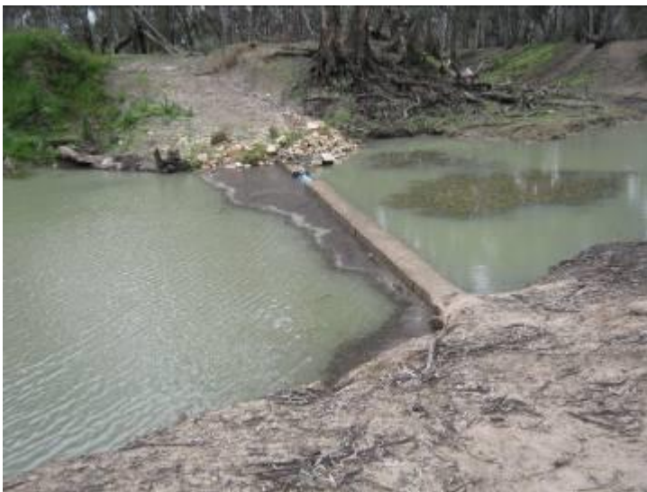
Narcooyia Creek Weir
