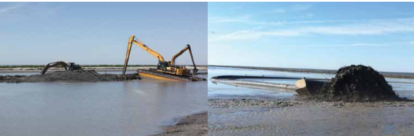
TE-48 Raccoon Island back barrier marsh creation project which enlarged the island by 53 acres. (Isle Dernieres Refuge)
