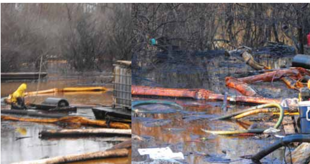
Bayou Sorrel oil spill (cleanup crew operating drum skimmer and oil impacts).
