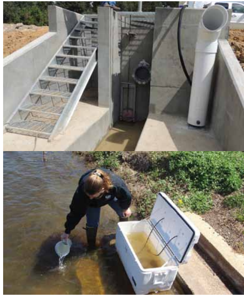
TOP: Huey P. Long Fish Hatchery's new harvest kettle/drain structure with water and air supply. BOTTOM: Florida largemouth bass fry hatched at Booker Fowler Fish Hatchery being released into a rearing pond at Natchitoches National Fish Hatchery (photo courtesy of Jan Dean, USFWS).
