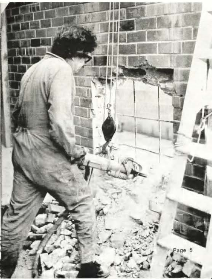
BELOW — Burley Griffin believed, amongst other things, in making his buildings solid. That hole represents two hours work with the jack hammer.
