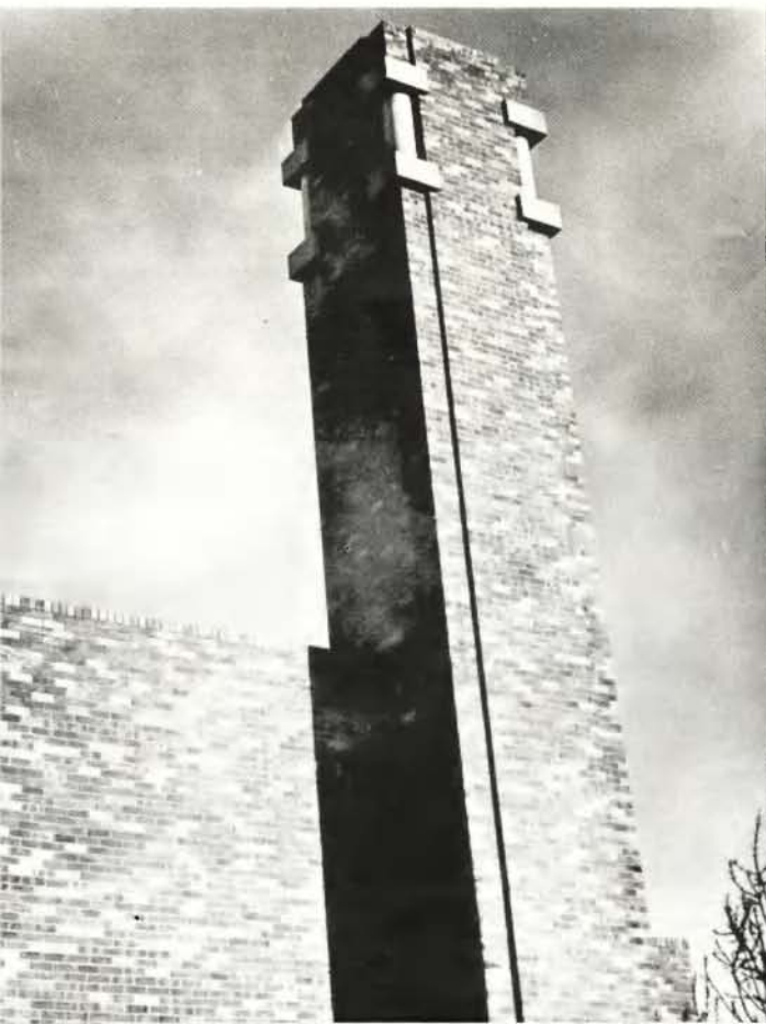
BELOW — The chimney at Thebarton, shortly due to be topped with beams for 20 metres and higher.
