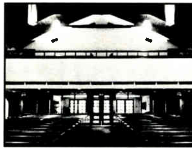
Balcony front before treatment
