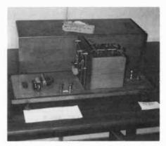
Another contest entry — this pre-1910 German coherer made by Kohl. Note the box with batteries to the right of the detector.
