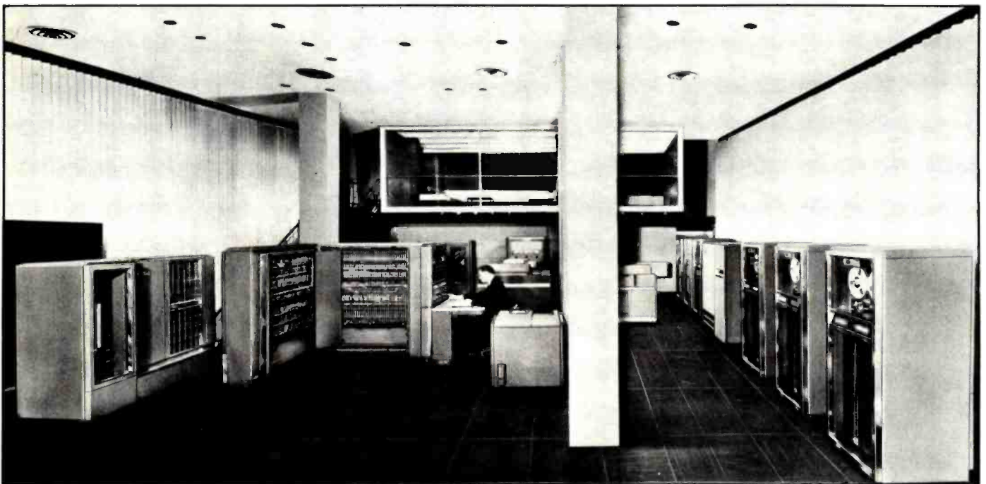
Photo 8: The IBM 704 had a core memory capacity of 32 K words with 36 bits per word. Although a card reader, punch, printer, magnetic tape drives and drums and a video display were available as peripherals, the concept of simultaneous IO and processing was not yet developed.
