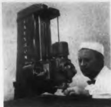
The Talyrond, a super-accurate measuring device, is used by Barden as a development tool; as a standard for correlation of other quality control instrumentation; as a gage for ultra-precise bearing parts. It measures roundness and waviness to five millionths of an inch.
