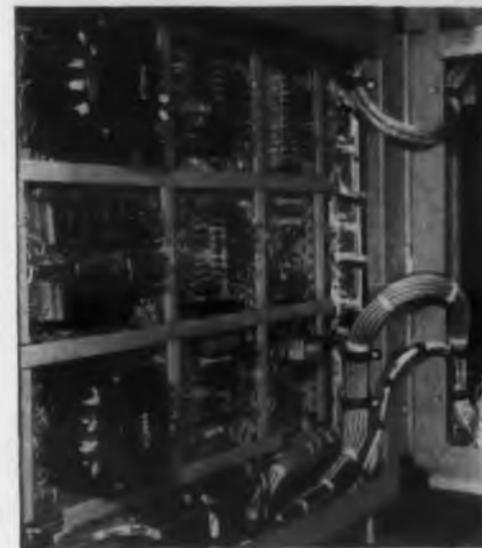
So easy to use—you just lay your wires in the duct, put them through holes to terminals, then snap on the cover—FAST and EASY. No wasting time with cover screws, hinges or mounting brackets. Speeds up production; eliminates costly time-consuming lacing, flat wiring or bundling. A cinch to maintain! Taylor Wiring Ducts are non-combustible, warp-resistant, acid-resistant, light in weight yet durable and rigid.
