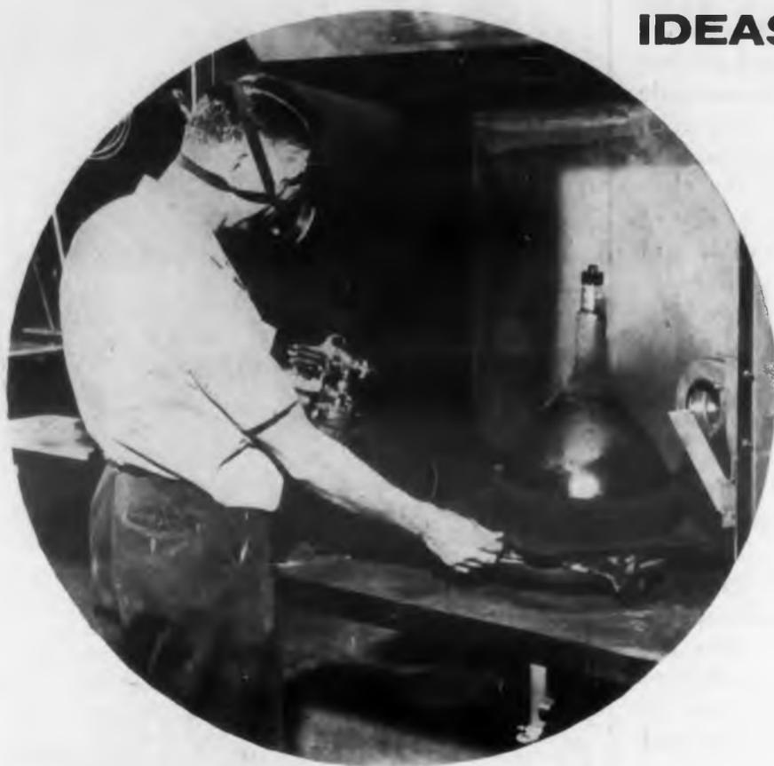
**Television tube** being sprayed with "dag" colloidal graphite. For exterior use the graphite is dispersed in lacquer, providing a smooth, black, adherent, conductive coating on any type of glass.
