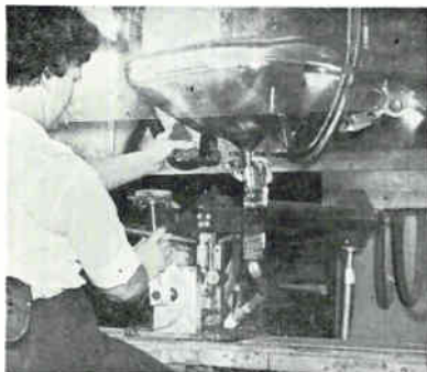
Getter flashing fixture moves with tube on conveyor
