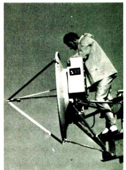
Link. For a CATV system test, technician adjusts 12-channel transmitter mounted on four-foot parabolic antenna
