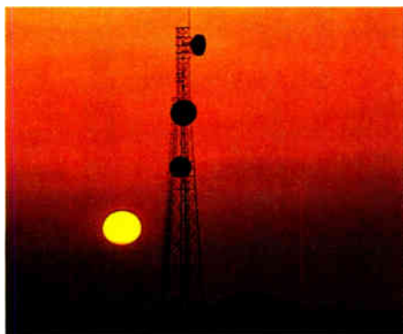
A microwave communication repeater station in operation at Mrassas, Libya.
