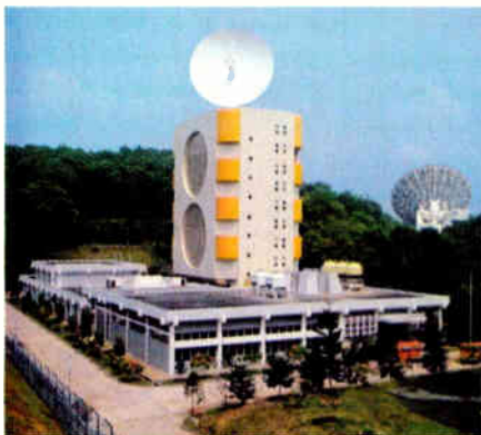
The C/L dual band 13m diameter antenna, with an NEC-built INTELSAT Standard A earth station antenna in the background.
