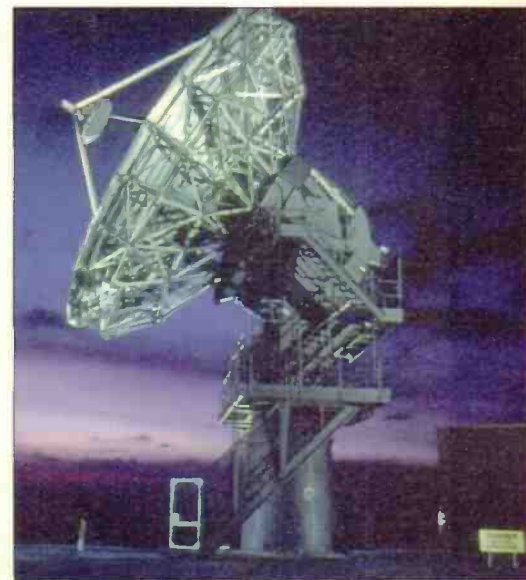
The BT coast earth station at Goonhilly, Cornwall.
