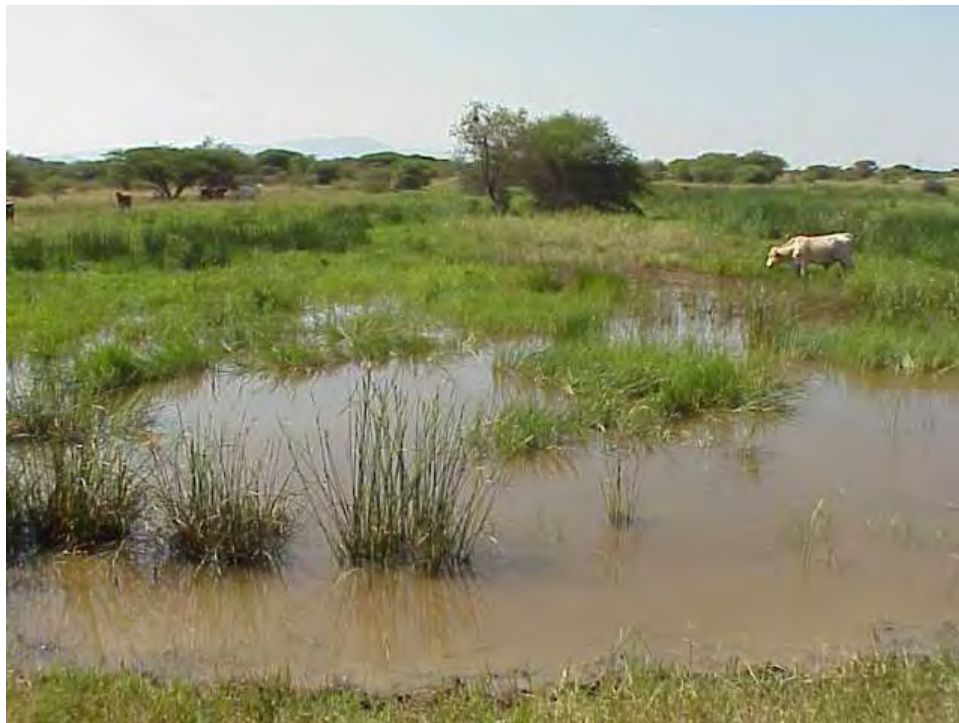
Figure 1.17: The impoundment at Haakdoorn – a spill over was constructed in the two-meter high earthen wall, which retains a large quantity of the flood water.
