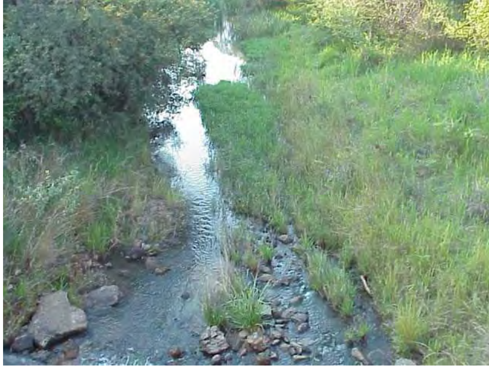
Figure 1.29: The Bad-se-Loop site, showing the river downstream of the road bridge.
