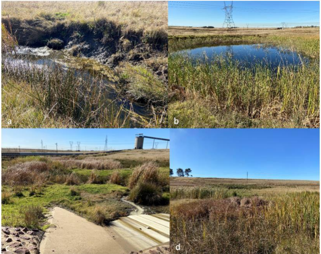
Figure 7-63 - Impacts: a) Soil Erosion at CVB main channel; b) pooling of water in dam; c) effluent discharge into the wetland; d) crop farming and cattle grazing in the wetland
