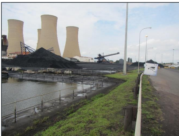
Figure 7-25: The completely transformed coal deposit area at Komati Power Station
