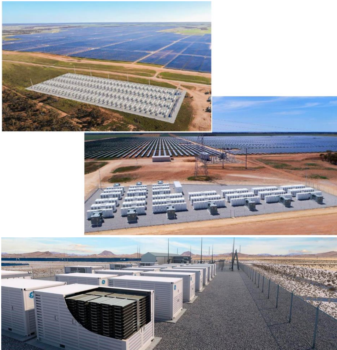
Figure 4-3 – Images of Typical BESS Systems
