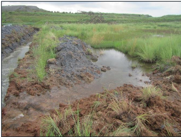
Figure 7-45 - Drainage channels that have been excavated by power station management to prevent the flooding of access roads
