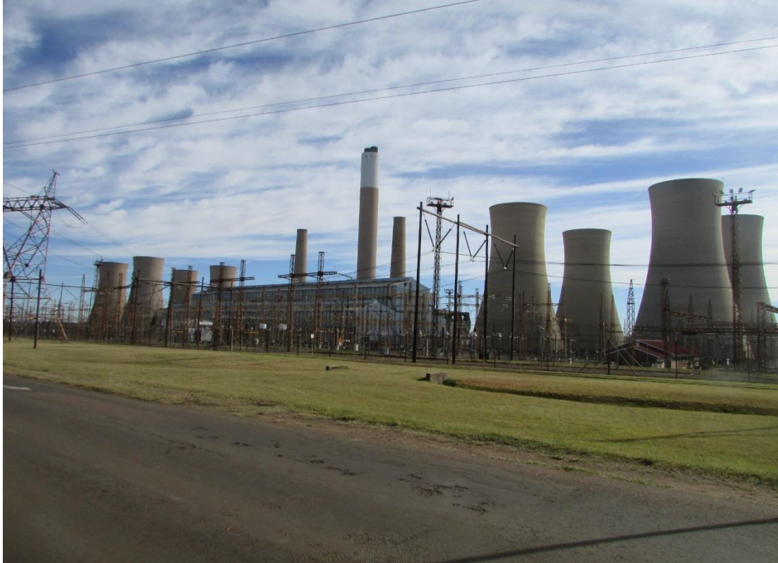
Figure 7-84: A view of the Komati Power Station (APAC, 2023)
