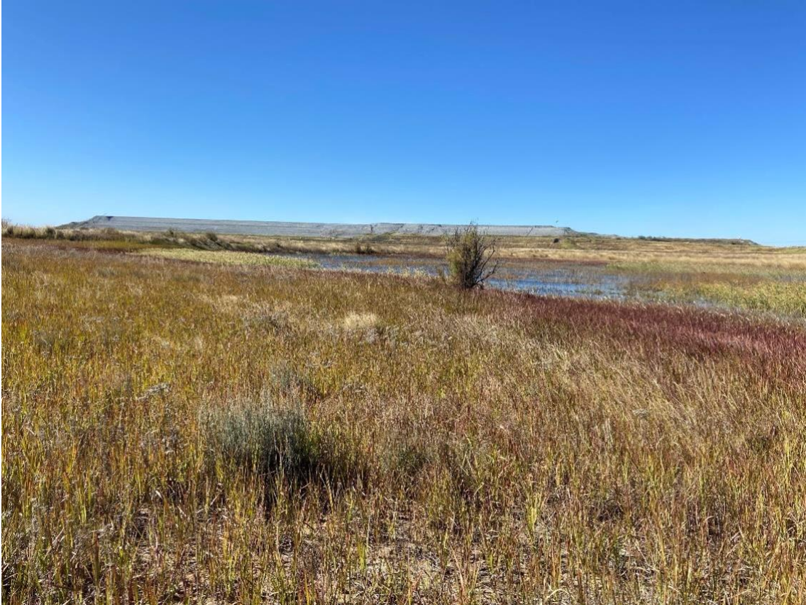
Figure 7-64 - Ash dam facility and pooling of water at dam
