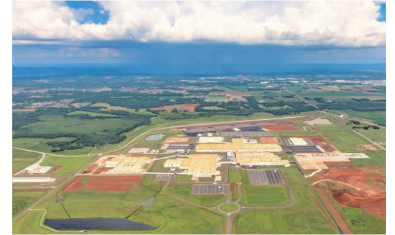
MTM, a new plant, in the U.S.A.
