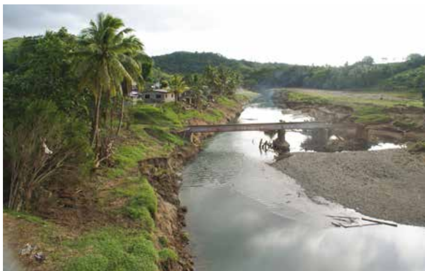
Infrastructure damage from cyclone Evan, Samoa
