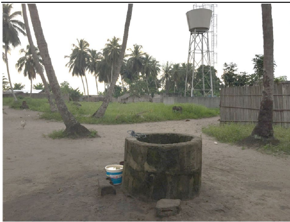
Figure 6.40 Water tower of Taboth
