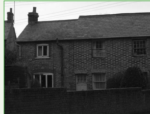
59-61 Carrington Hall Road
